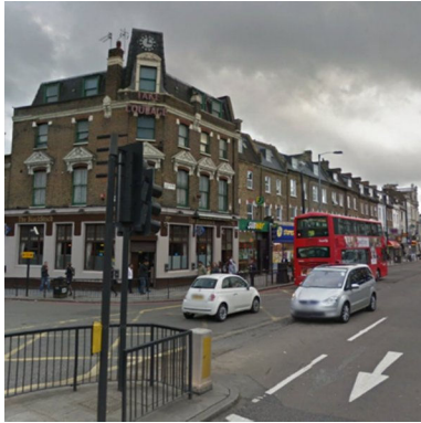
Photo 19: Intact historic block
