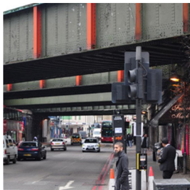
Photo 22: Seven Sisters Road viaducts
