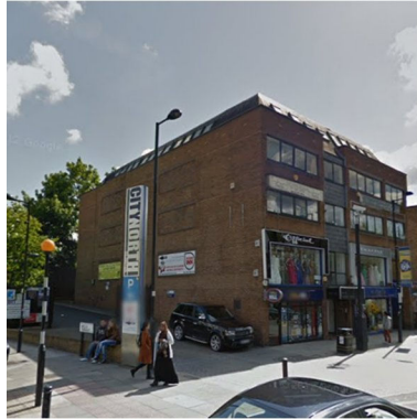
Photo 13: City North site
