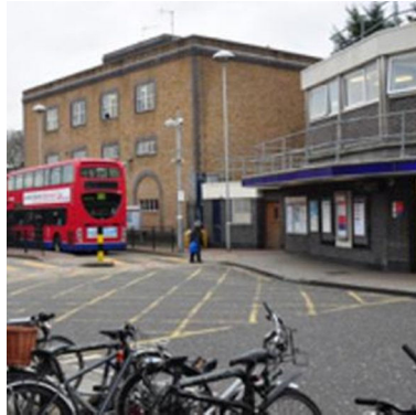
Photo 14: Northern station entrance
