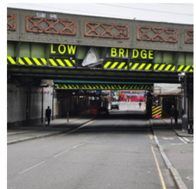
Photo 12: Bridge, Stroud Green Road
